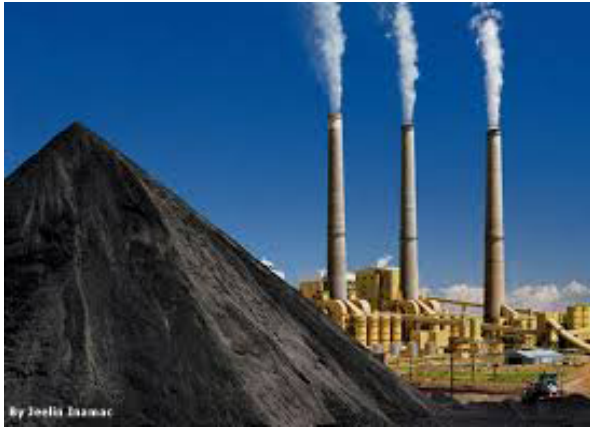
Figure 5 - A Coal-Fired Power Plant
