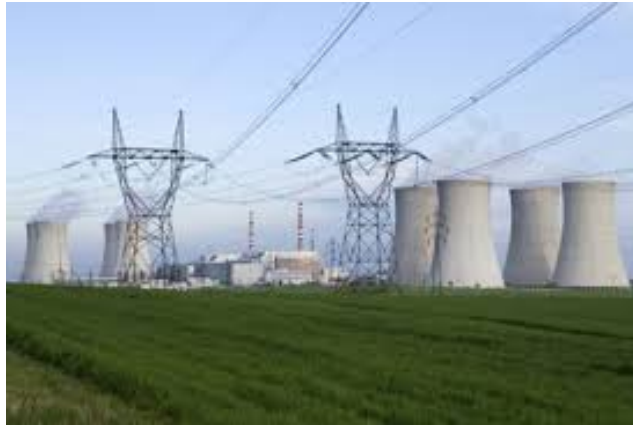
Figure 9 - A Nuclear Power Plant with Water-Cooling Towers and the Beginning of the Electrical Grid in the Area.
