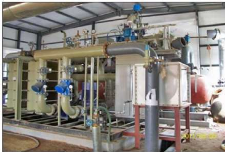
Figure 5. Geothermal power generation system: binary expander.
