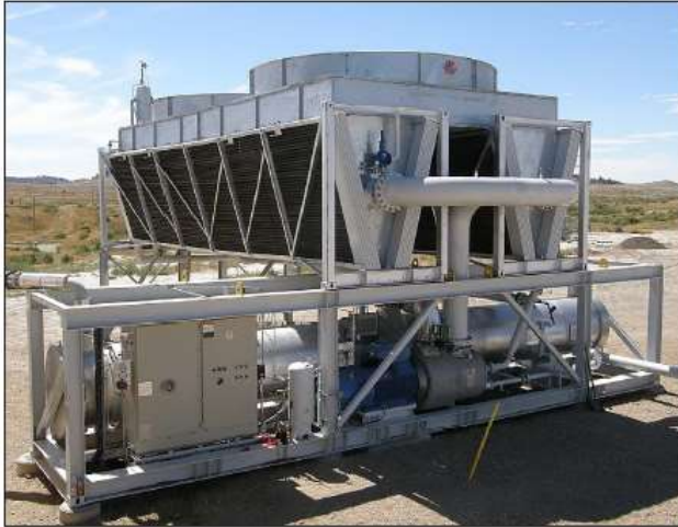
Figure 1. The RMOTC OEC, commissioned in September 2008.
