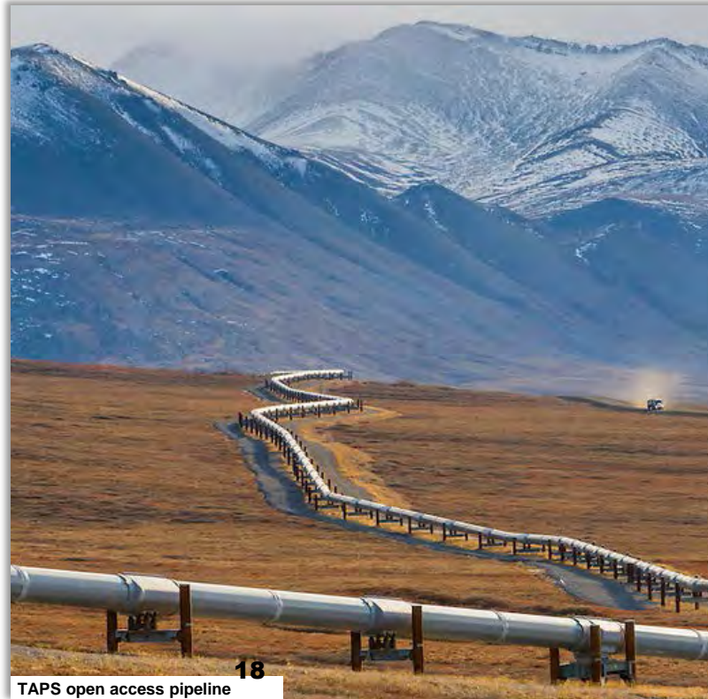
TAPS open access pipeline 18
