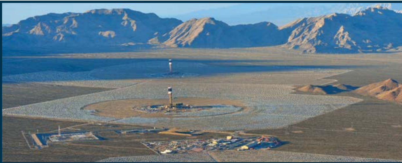
This aerial photograph is of the Ivanpah Solar Electric Generating System in California's Mojave Desert, at the base of Clark Mountain. Photo courtesy of Michael Collier.
