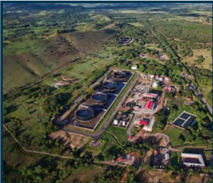
Modern facilities for oil production in eastern Llanos.
