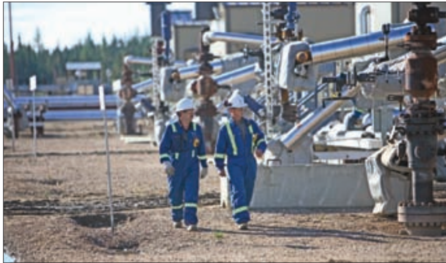
A closer view of operations at the Christina Lake heavy oil operation in Canada; (left) an insulated pipe and emergency shut-down valve for the field's SAGD operation in northeast Alberta, which is constantly being checked (right) for potential snags.
