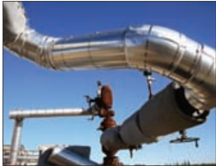
A closer view of operations at the Christina Lake heavy oil operation in Canada; (left) an insulated pipe and emergency shut-down valve for the field's SAGD operation in northeast Alberta, which is constantly being checked (right) for potential snags.
