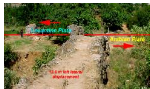
Href aqueduct, 13.6 m offset through three seismic events offset
