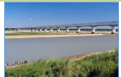
Irrawaddy Bridge, Magway
