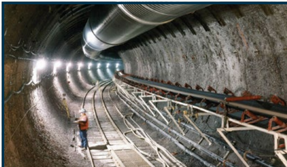
The underground exploratory studies facility is located at Yucca Mountain in Nevada. It was built by the Department of Energy to determine if the location was suitable as a deep geological nuclear waste repository. Courtesy of the Department of Energy.
